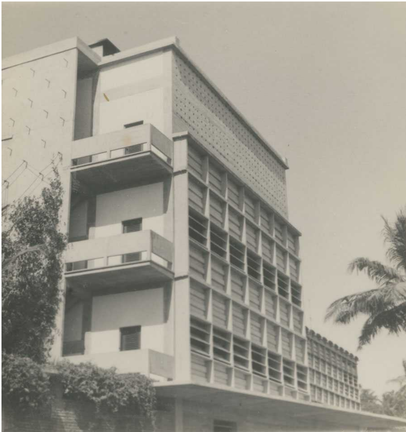
North elevation of centre & west
