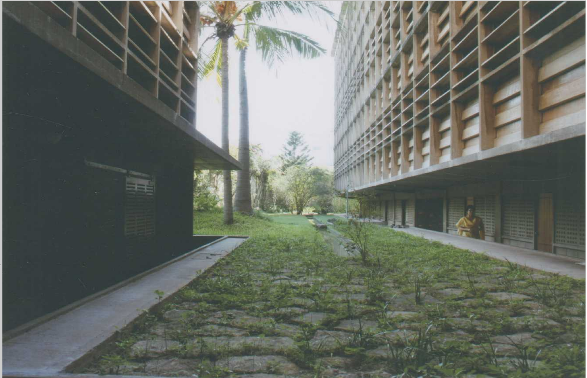
North East elevation & east service corridor. Boiler room on left
